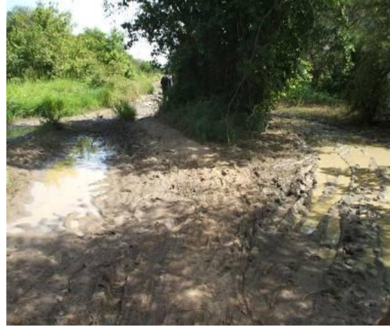
Figure 9: Muddy Tracks in the Road (Davis 2007)
